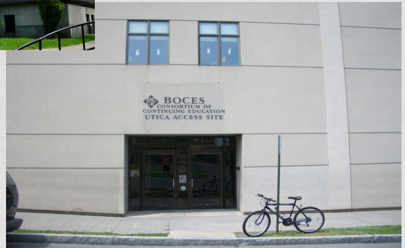
Utica ACCESS Site 508 Second Street
